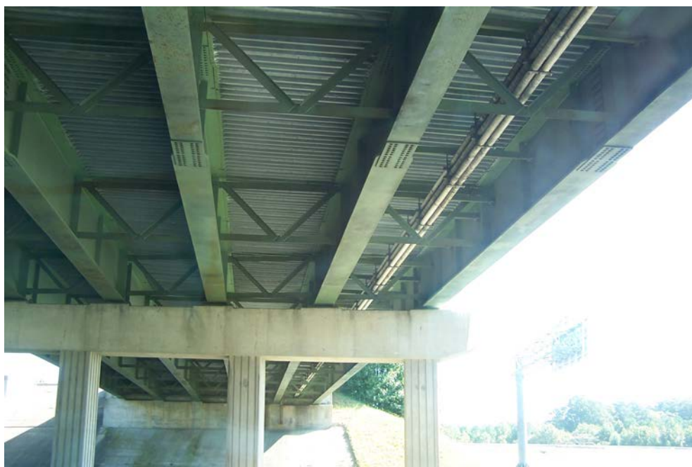
Figure 3: Existing Conduit on Bridge Crossing
