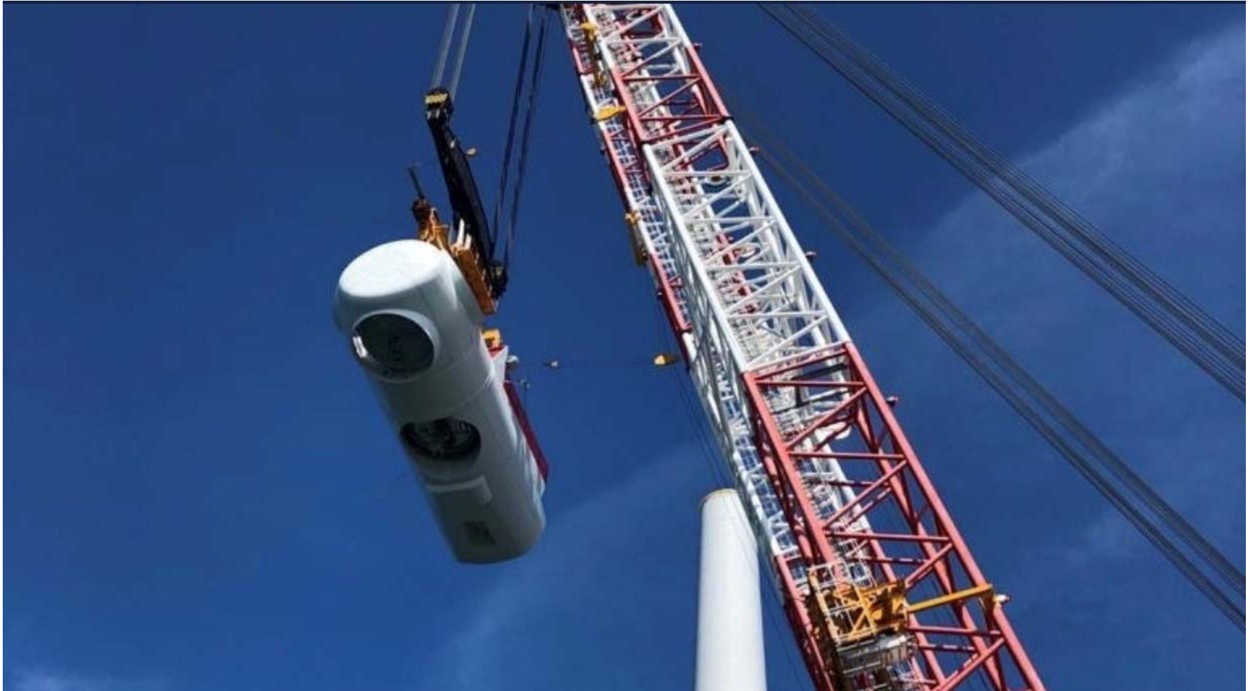
Nacelle installation
