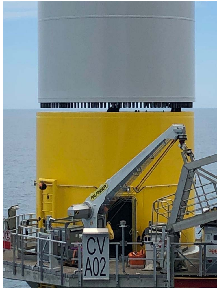
Tower installation
