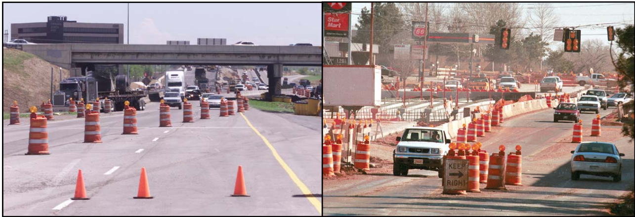
PICTURE 4 – Construction areas create conditions that can be extremely hazardous to drivers and highway workers. Adequate signage, warning devices, and barrels and cones help minimize hazards and safely direct traffic.
