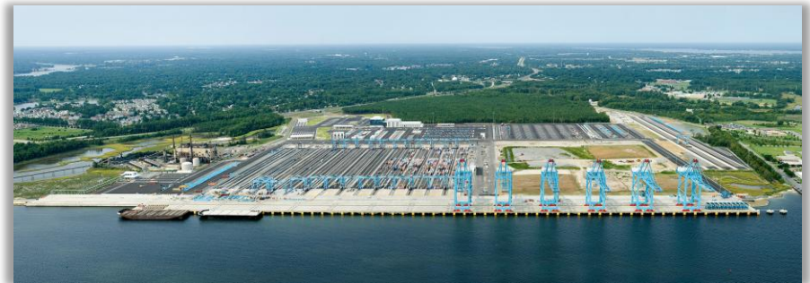
Aerial View of APM Terminals Virginia located in Portsmouth
