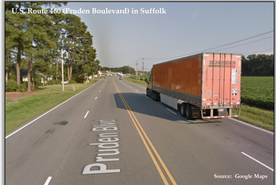
U.S. Route 460 through the City Suffolk, Isle of Wight County, Windsor, and Southampton County has 10 foot lane widths.
