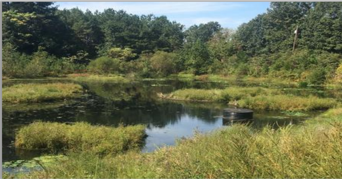
Figure 1: Floating Treatment Wetlands in a Stormwater Pond
