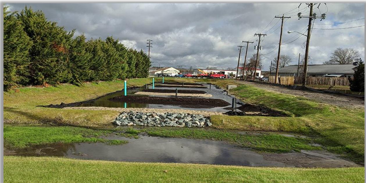
Figure 14: Submerged Gravel Wetland located in the Town of Berlin, Maryland
