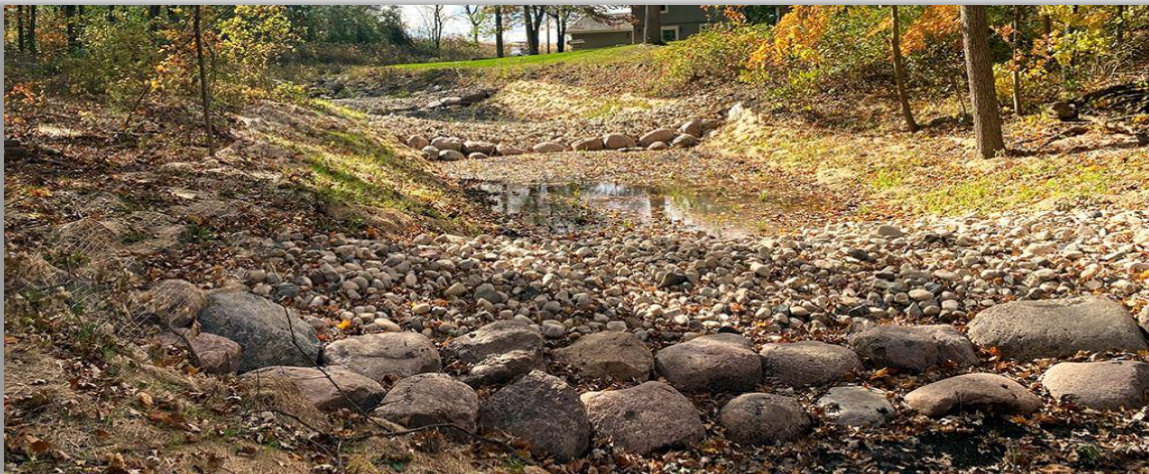
Figure 20: An Example of a Regenerative Stormwater Conveyance System
