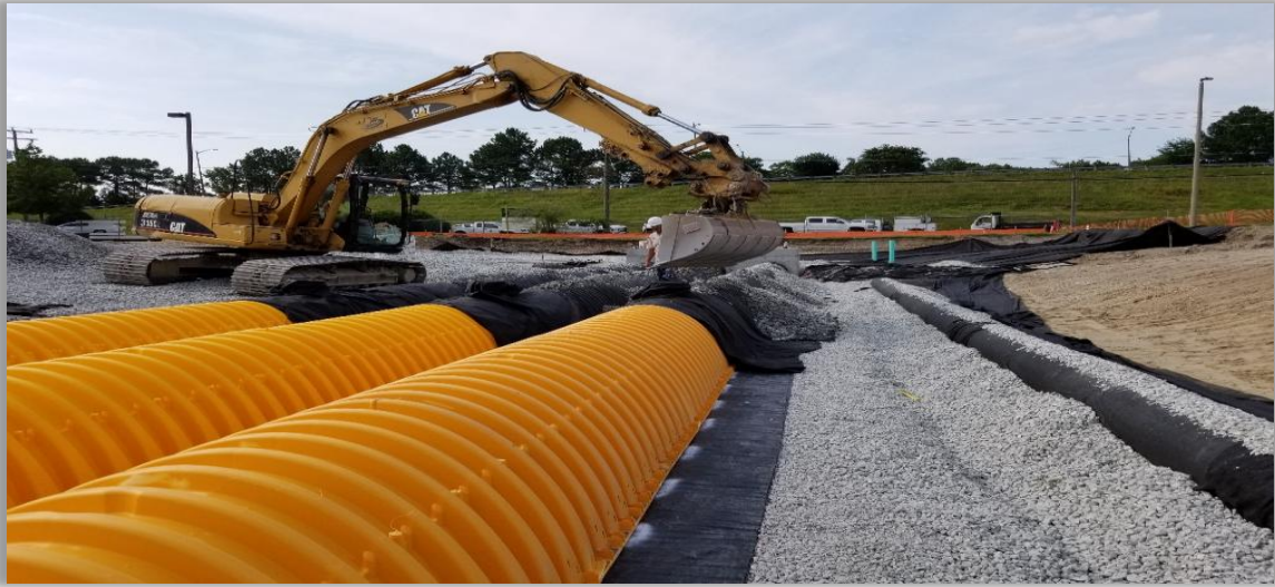
Figure 18: An Example of an Underground Storage BMP
