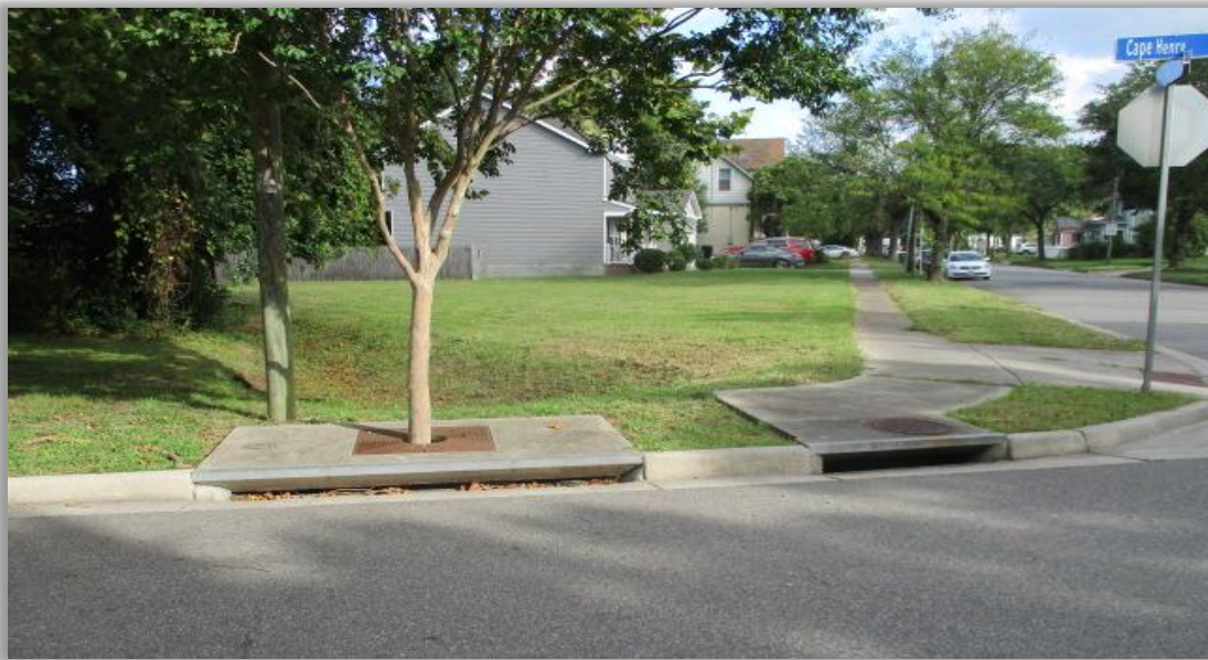
Figure 16: An Example of a Filterra System
